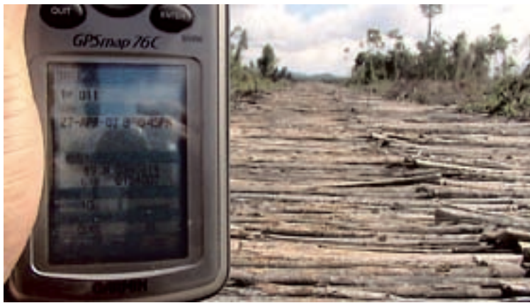
Figure 12. Road in the PT ANI area constructed with swamp forest logs (April 2006).
